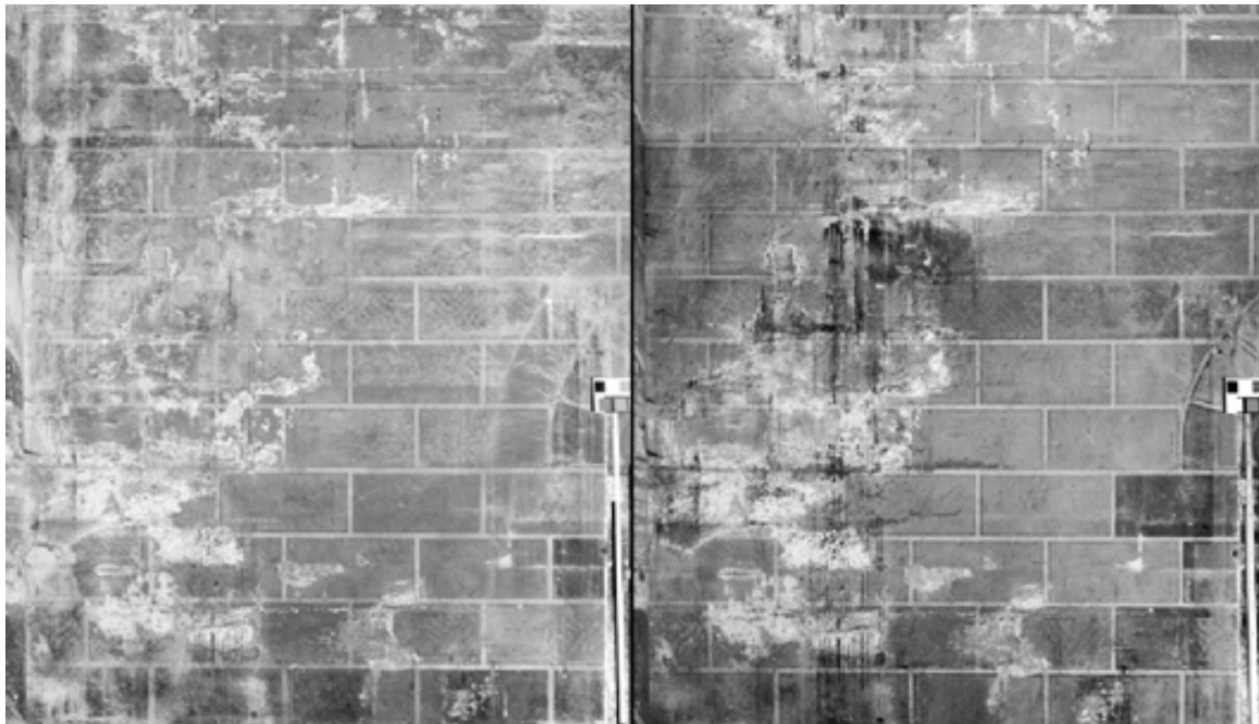
Detail of the north wall in infrared band (left) and UV band (right). The infrared band suppresses the visualisation of the cement. The UV band enhances this contamination
